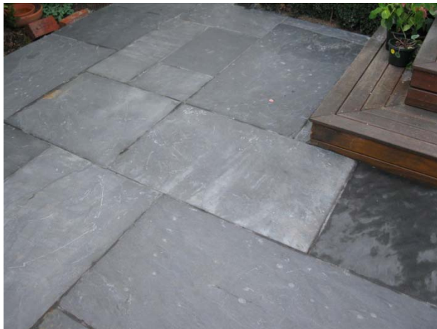
Large Ashlar Paving
