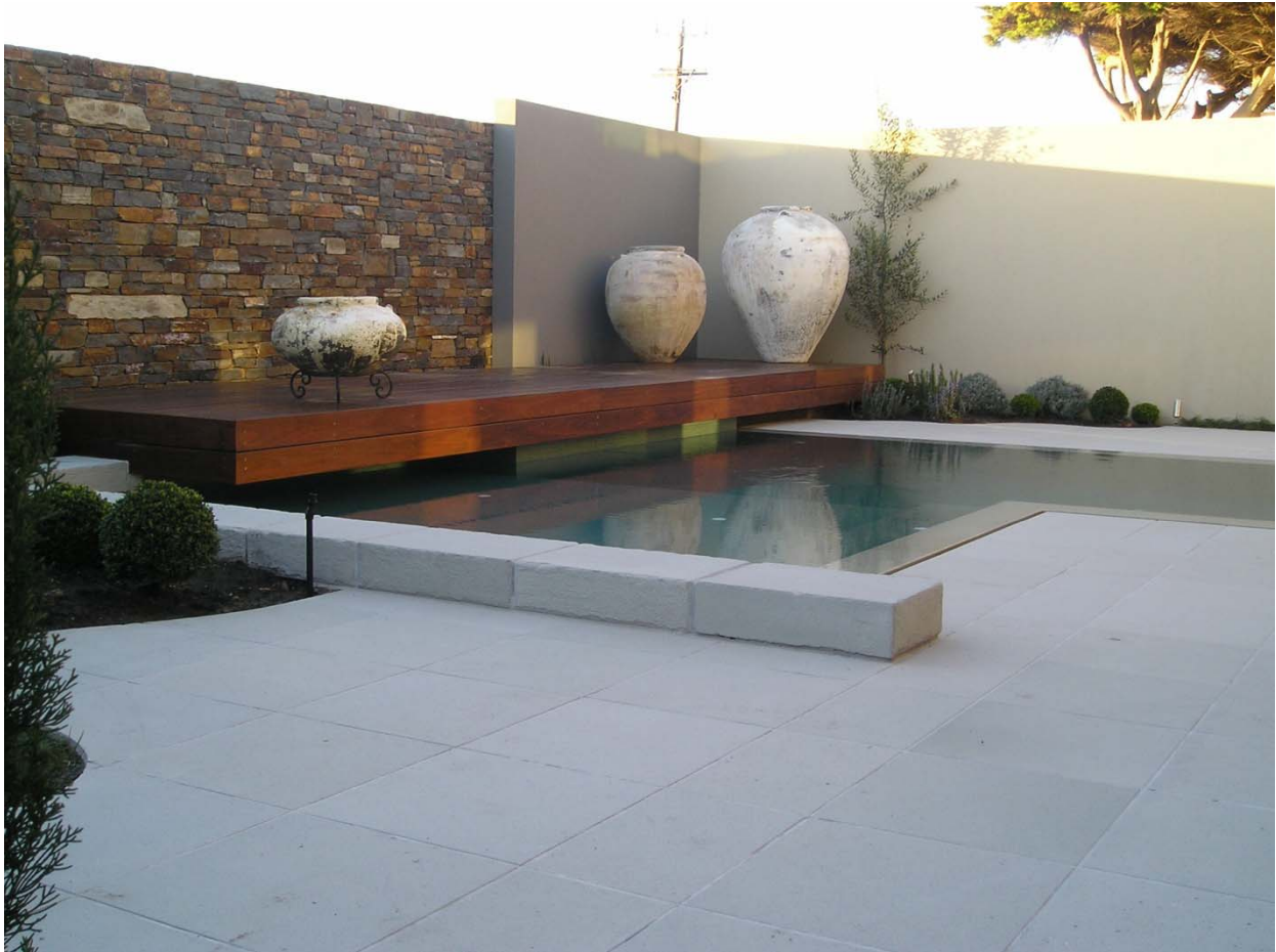
Sandblasted Paving & Bush Hammered Blocks
