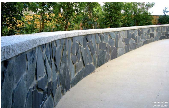
Monaro Stone Charcoal Cladding & Granite Capping
