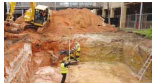
Area excavated to required dimensions.
