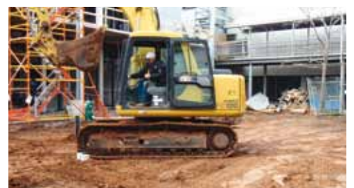
Completed installation under trafficable area.
