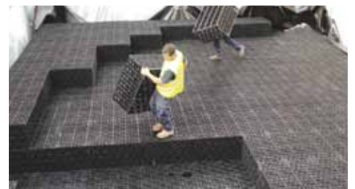
Assembled modules installed and enveloped with geotextile and membrane.
