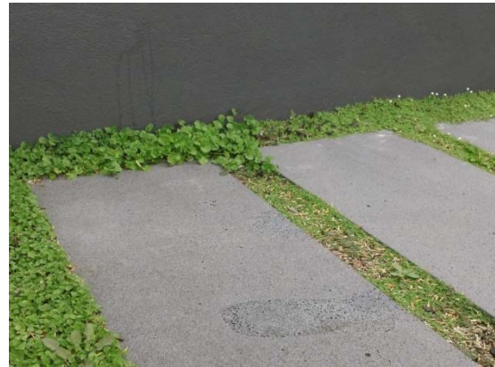
Diamond Sawn Paving
