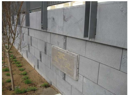
Diamond Sawn at St Kilda Town Hall
